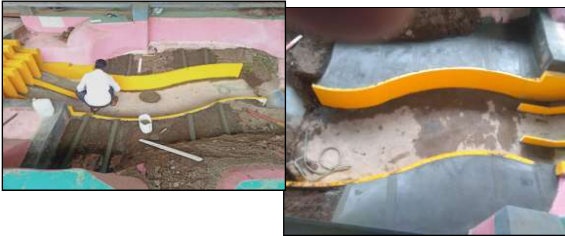
Photo 17 to 20 : Curved stilling basin EDA (work in progress)
